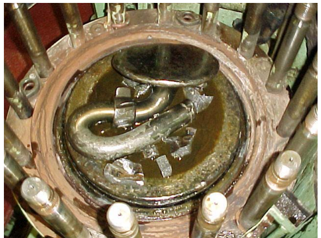
Fig. 117 Broken valve spindle curled-up in the compression space. (Author)
