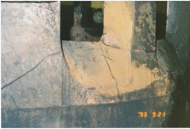
Fig. 97 Cracked cylinder liner, KSZ90BL. (Author)
