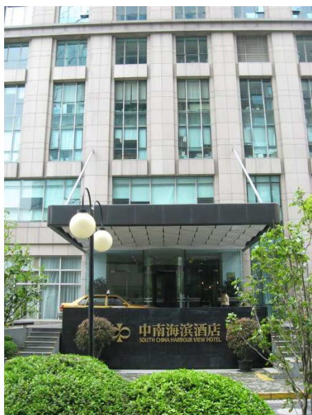
図1, Shanghai South China Harbor View Hotel
